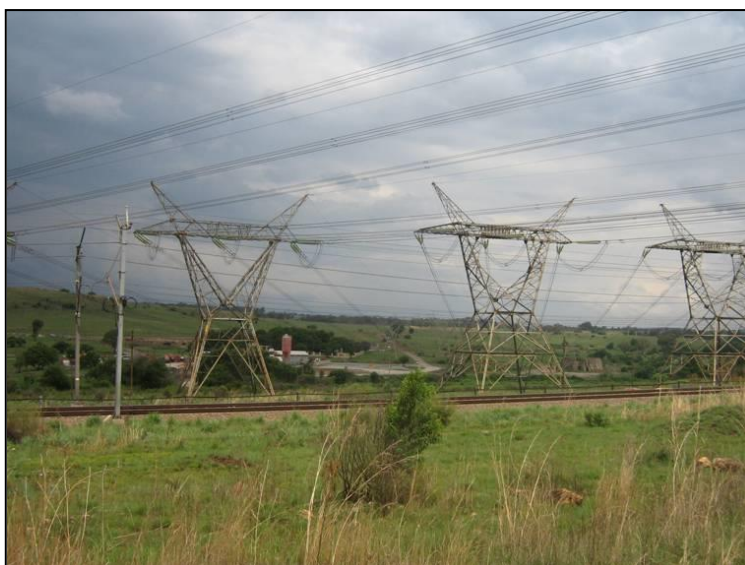
Figure 12: Land use surrounding the proposed route corridor section through the CTMM
